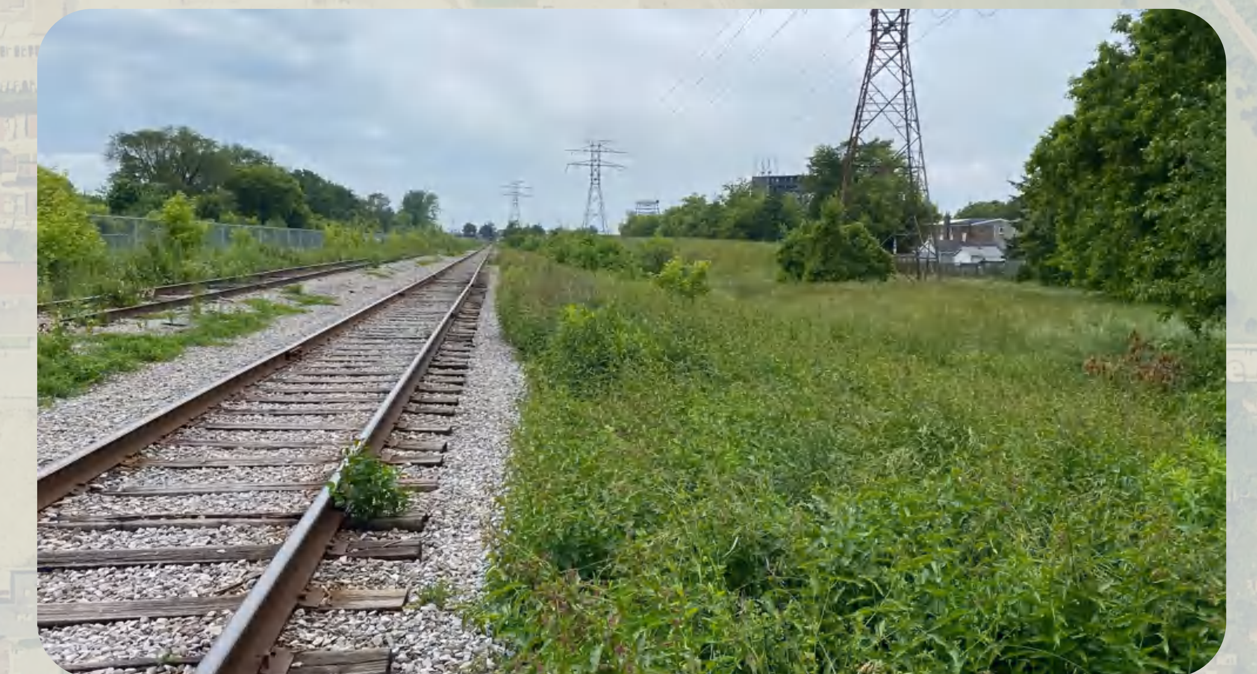
Facing south-west along the rail corridor
