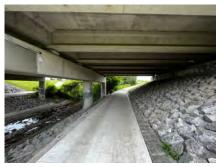
Figure 6. An existing underpass allows grade-separated crossing of McNicoll Ave on both sides of the river. There is a lack of lighting fixtures in the underpass, so while during the day the underpass is sufficiently lit, it may be dangerous at night. (Photo by: Anastasiia Ostrovskaia)
