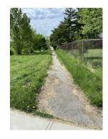
**Figure 45.** Path beginning at Middlefield Rd with uneven surface and poor maintenance. (Photo by, Karen Khan)
